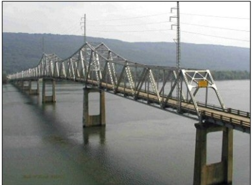
Cantilevered through truss bridge over Tennessee River on AL 35 at Scottsboro is 2143 feet long. Built in 1930, it is still open to traffic
