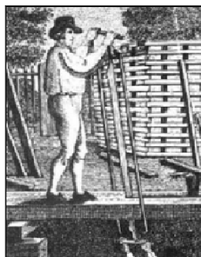
A "saw pit" (or "sawpit") is a pit over which felled trees are placed so two men, one above and one below, may use a long two-handled pit saw, often called a whipsaw.
